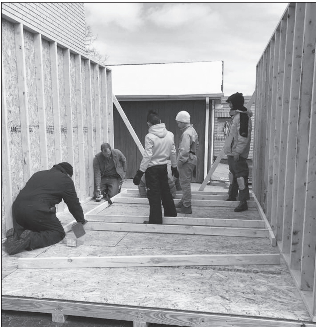
Joe Rohde, son of Jeffrey and Bridget Rohde of Steubenville, and 25 volunteers including members of his family, build a storage shed at Bishop John King Mussio Central Elementary School, Steubenville. Joe is building the shed as his Eagle Scout project from Troop 401. A freshman at Catholic Central High School, Steubenville, Joe is a parishioner of Holy Family Parish, Steubenville. Mike Homol, Homol Construction Inc., supervised the project. (Photos provided)
