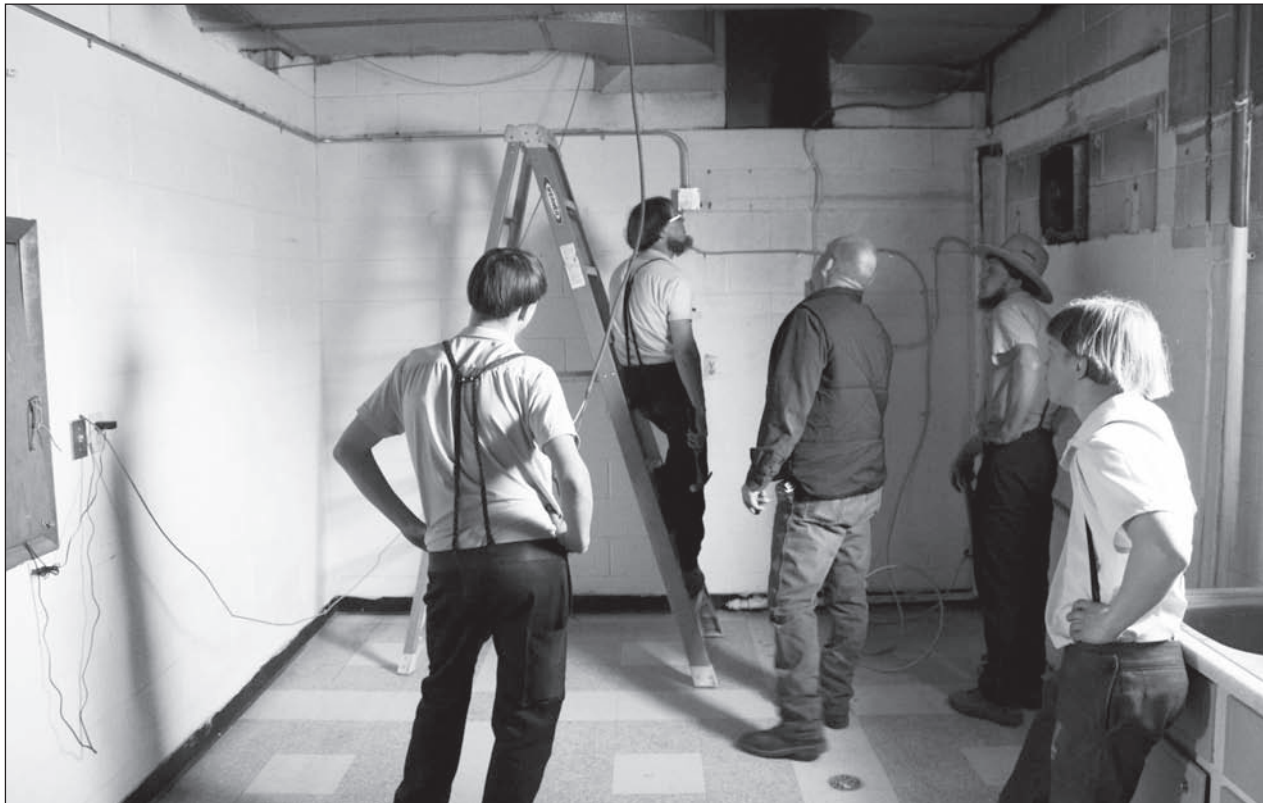
D. Scott Yarman Contracting of Cadiz work in the lower level of the Sacred Heart Center of Hope, Steubenville. Renovations at the 430 Slack St. building began April 9. (Photo by DiCenzo)
